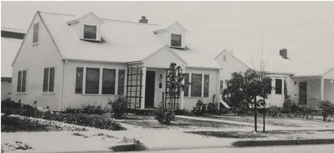
Figure 1. 516 G Street (left) photographed in 1943 (Lofland and Haig, Images of America: Davis 1910s-1940s , photograph credit Clarence Barry)
